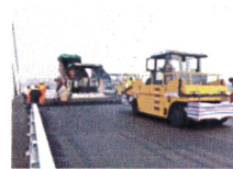
Paving of KT-BEP
